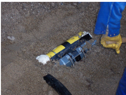
Mounting of the mechanical protection
