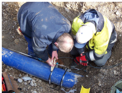
Installation of the sensors
