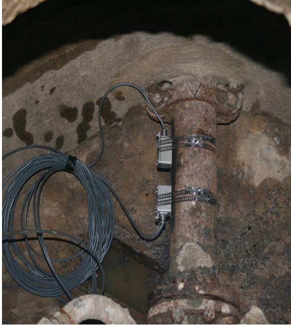
Figure 3 installation of LeakControl in a manhole
